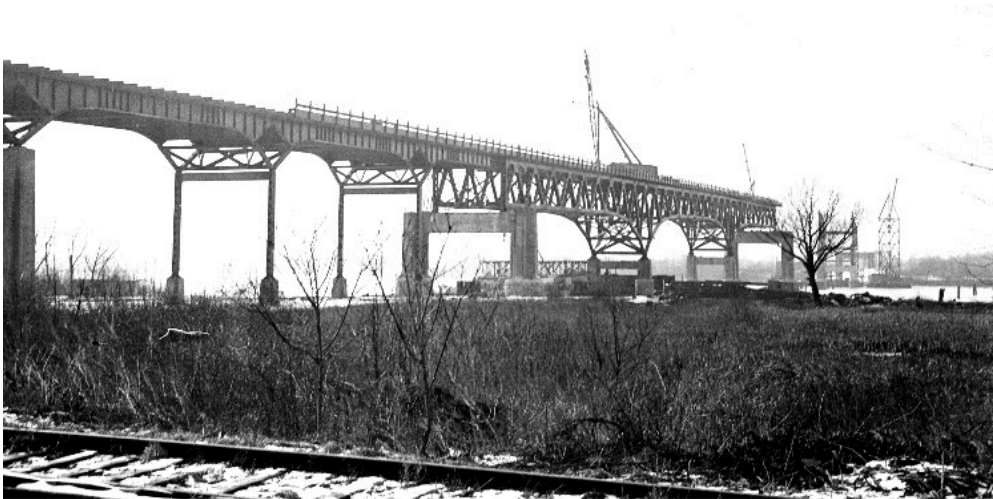
Construction of the Susquehanna River Bridge 1906
