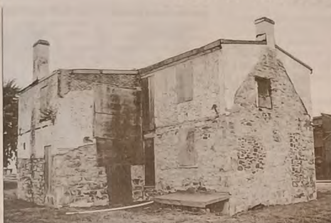
If you look closely, the layers of remodeling can be seen. The first layer (bottom) of stone shows the original building of 1827 – a small rectangle with the kitchen off the back. The next layer (white) shows the raised roof over the house and kitchen done in 1884. In the 30s the L section (kitchen) was raised to match the roof line and an addition was created (can't be seen) to make the building a rectangular shape. photo courtesy of Bobby Parker
